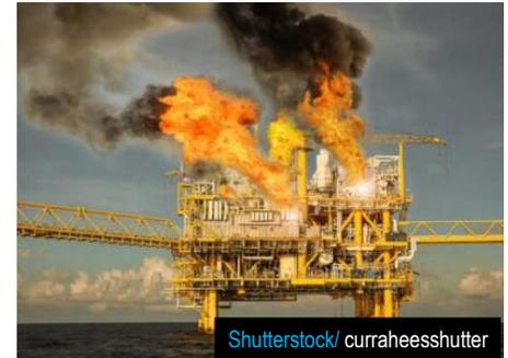
*Flaring the excess methane from an offshore oil and natural gas well.*
