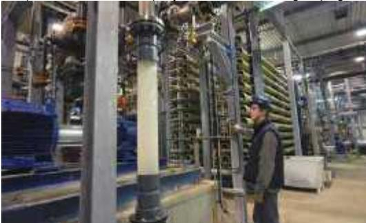
*Dow's Terneuzen plant in the Netherlands accepts 10,000 cubic meters of municipal household wastewater each day, has it purified by the water company, and uses it to generate steam and feed its manufacturing plants.*
